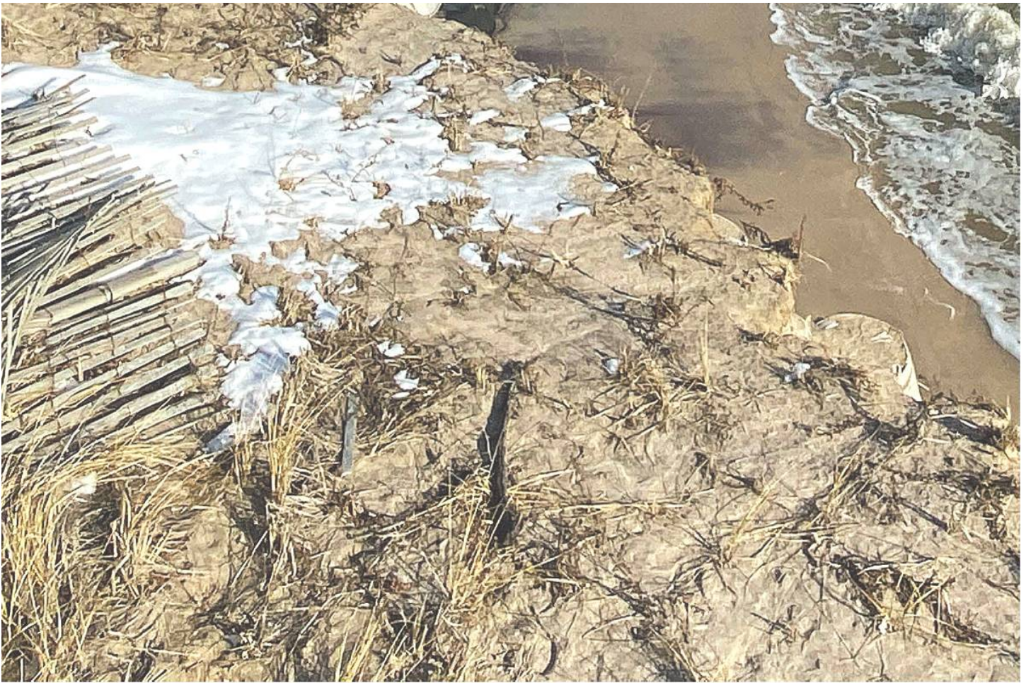
Geocubes are exposed at Quogue Village Beach after a winter storm. DANA SHAW
